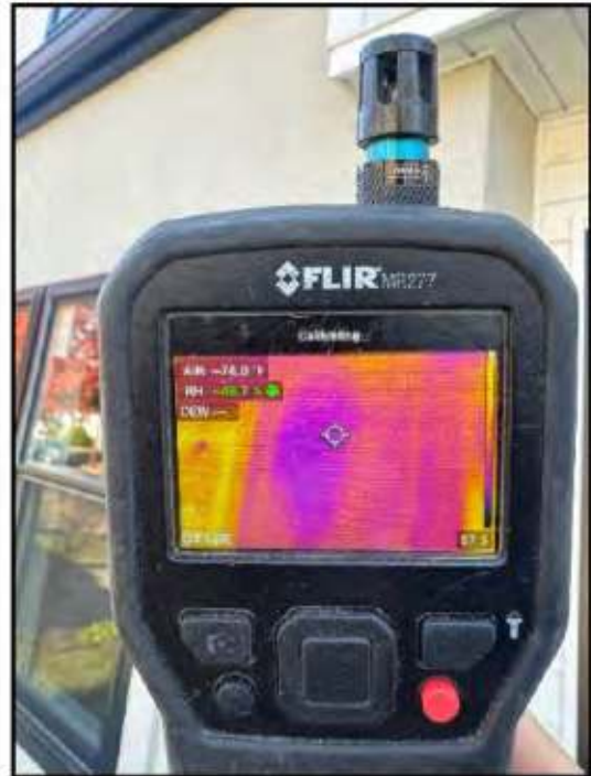
84. Possible water infiltration behind EIFS
