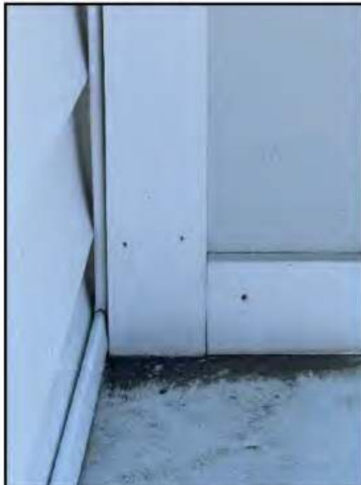
71. Exposed fasteners
