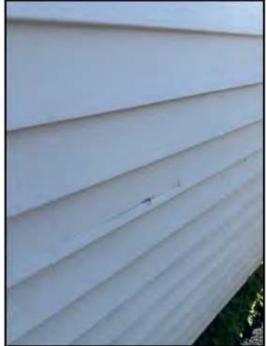
73. Mechanical damage
