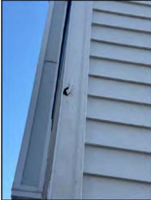
72. Mechanical damage
