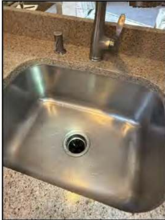
235. Switch/button exposed on sink/countertop
