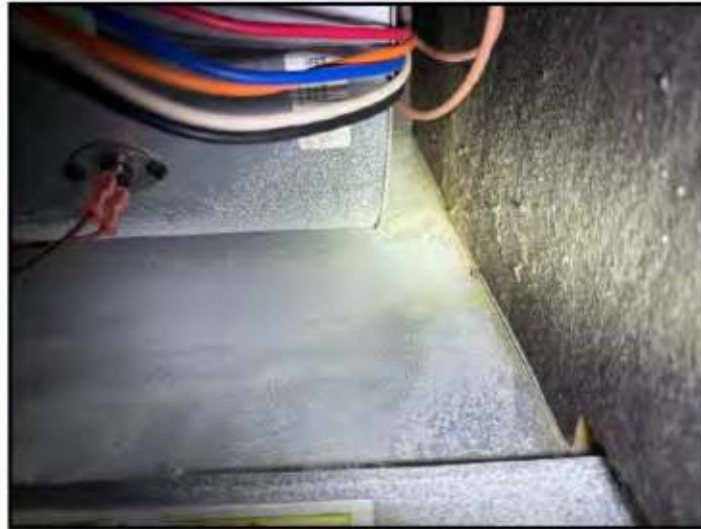
148. Rust / corrosion
