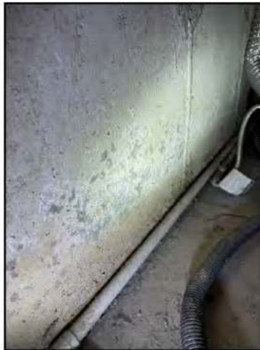
43. Efflorescence
