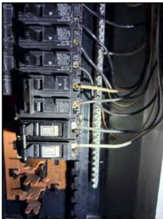
130. White wires connected to breakers not...
