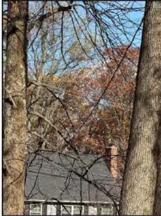
12. Branches / vines interfering with wires
