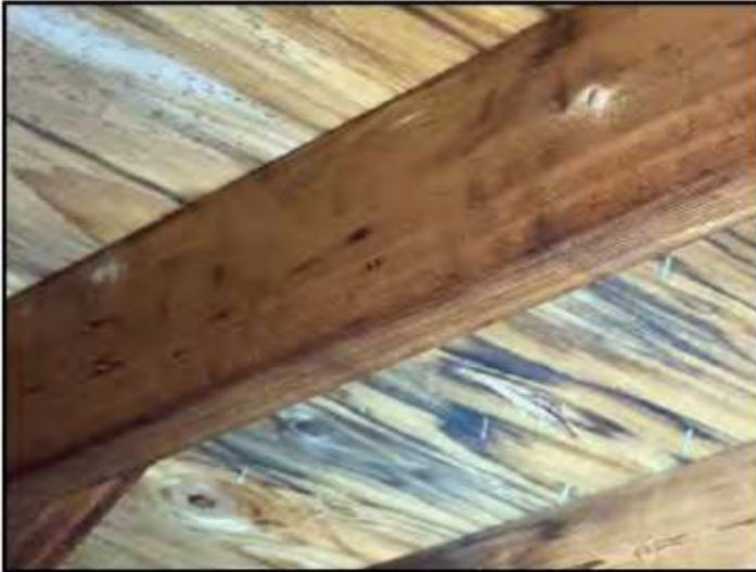
120. Water damage
