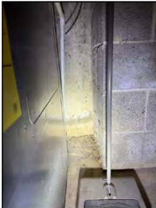
219. Efflorescence
