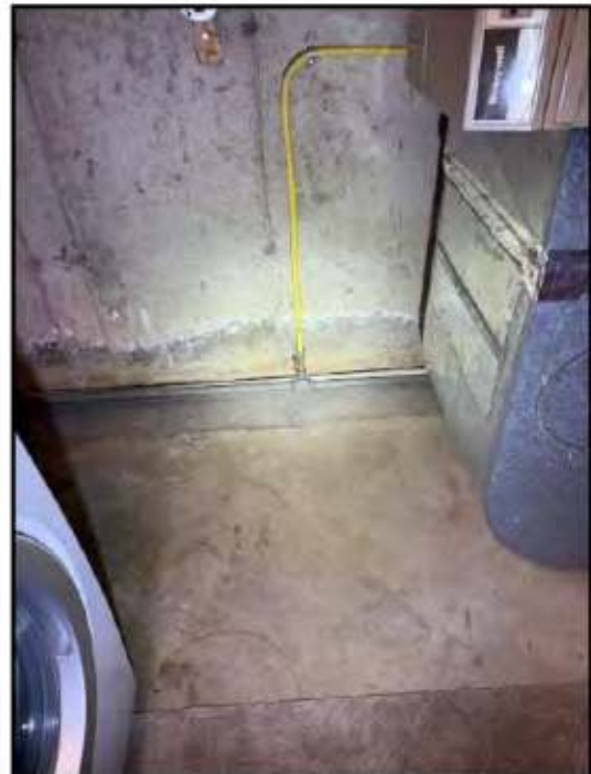
220. Efflorescence
