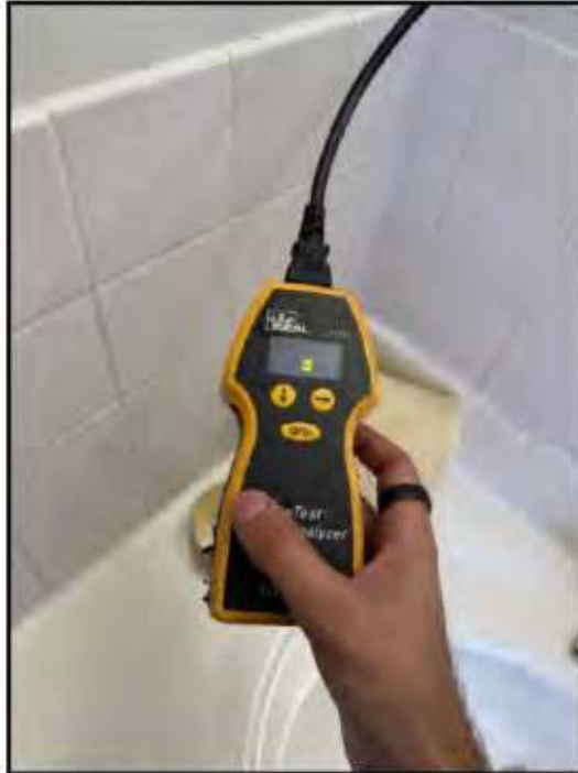
137. GFCI/GFI needed (Ground Fault Circuit...
