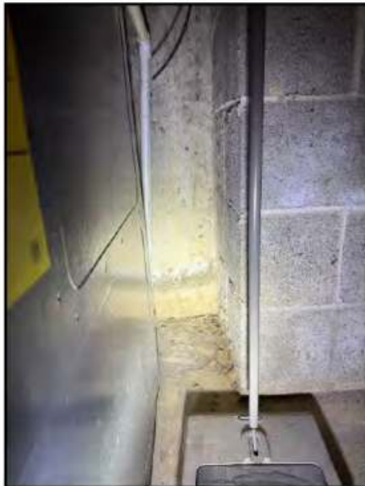
41. Efflorescence
