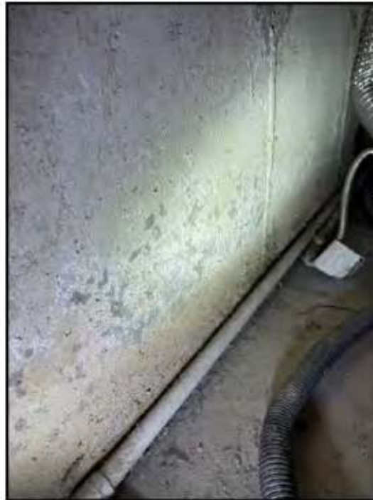
221. Efflorescence
