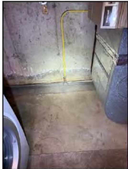
42. Efflorescence
